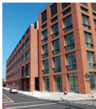
Water collected on the roof of the research building at 10 Amistad St. is used in ultra-low-flow lavatories and dual-flush toilets.
